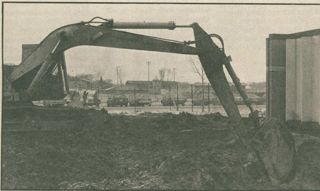
The foundation for the new classroom addition at the southwest corner of BHS was prepared by digging with a back hoe and then filling the hole with sand. (Photo by Paul Wilson)
