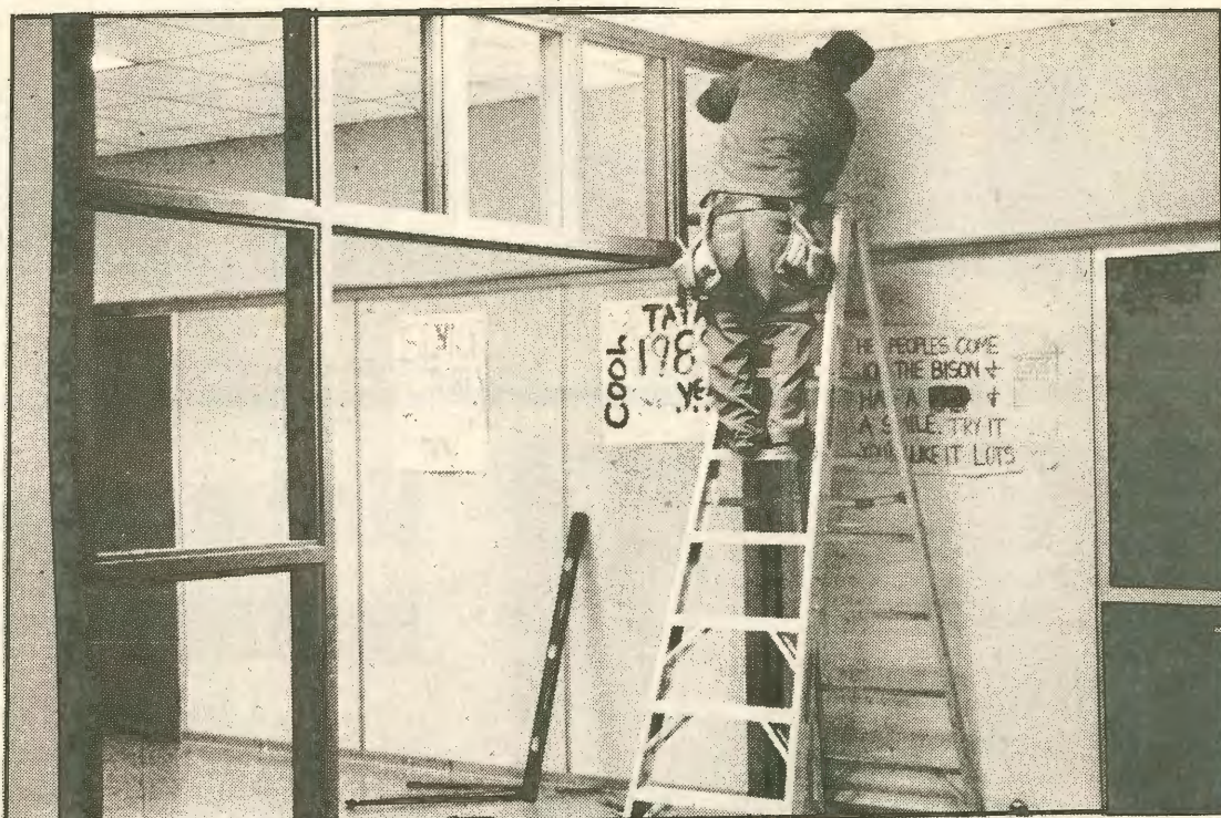
A Winkelman Building Corp. employee insists a fraction of the three million dollar renovations. The frame is part of a wall built to suppress lunch-time noise from the mall. (Photo by Paul Wilson)
