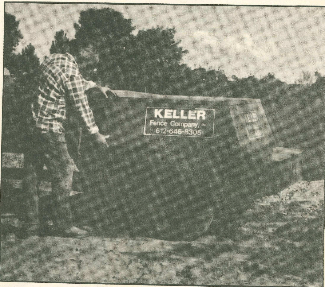
THE NEW TENNIS COURTS continued to be built as workers hastily tried to get them finished before the 1991-92 school year. Here, a construction worker starts up a high pressure air jackhammer as others pound fenceposts into the asphalt surface of the court. (Photo by Mark Ludwig)
