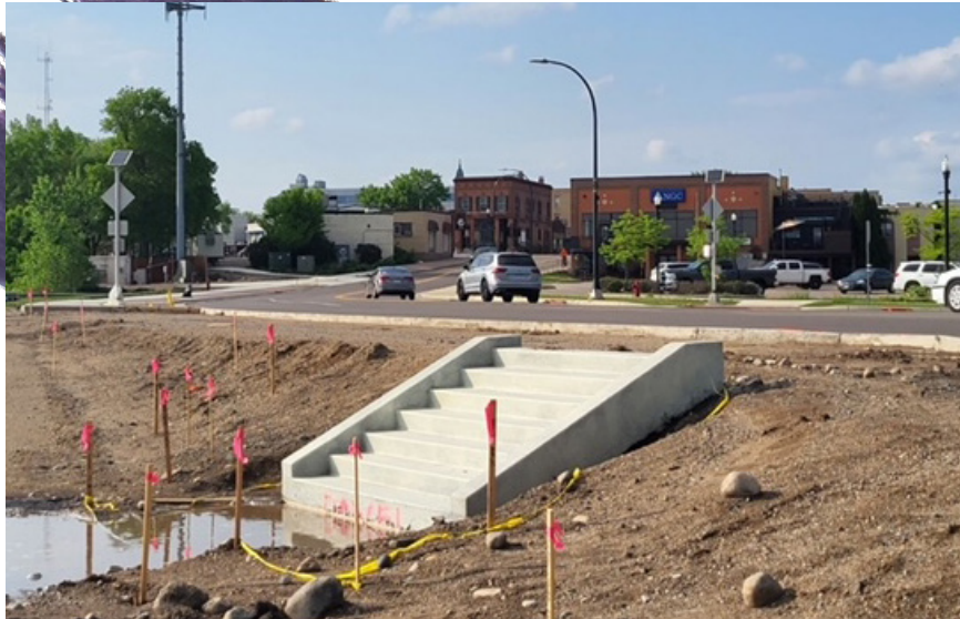
In-process downtown construction. Photo by Sirena Rygiel
